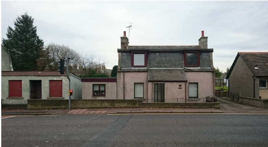
The view from Stonewood Road showing house, site access & original shop.
